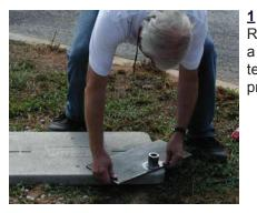
Remove lid and place on a level surface. Apply drill template directly over pre-drilled hole as shown.
