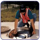
**Step 2**Set stainless steel pan onto manhole ring.
