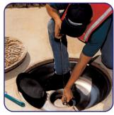
**Step 4**Hand tighten stainless steel nut on threaded rod and check clearance.
