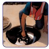
**Step 3**Raise ledger bar into position by pulling up on T-handle.
